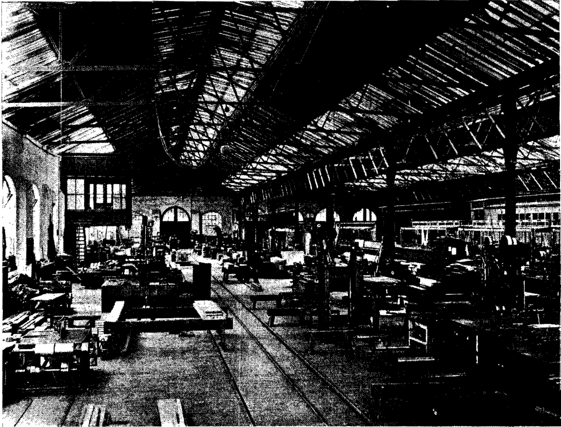
VICTORIAN RAILWAYS. CAR SHOP, NEWPORT.
