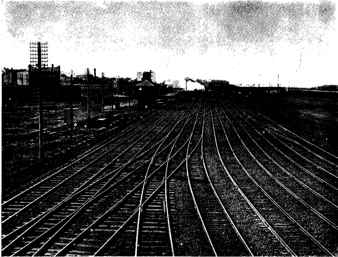
VICTORIAN RAILWAYS. NORTH MELBOURNE JUNCTION.
